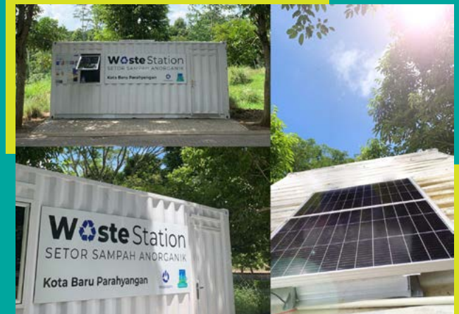
Rekosistem's waste station, equipped with solar panel
